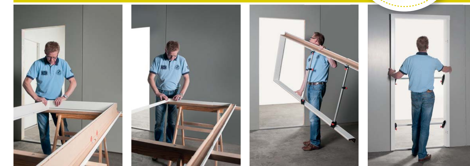
1. Assembler le chambranle.
