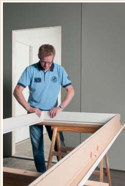
1 • Assembler le chambranle.
