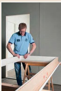
1 • Assembler le chambranle.
