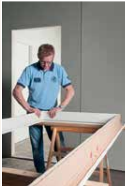
1 • Assembler le chambranle.
